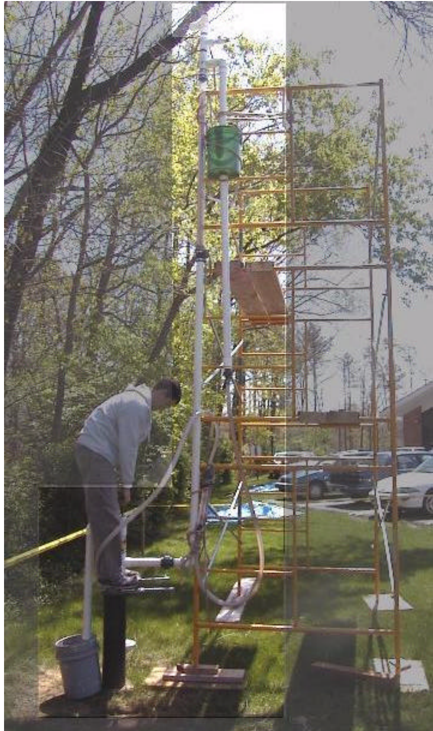
Figure 6 - Pump output and water return/dampening system
