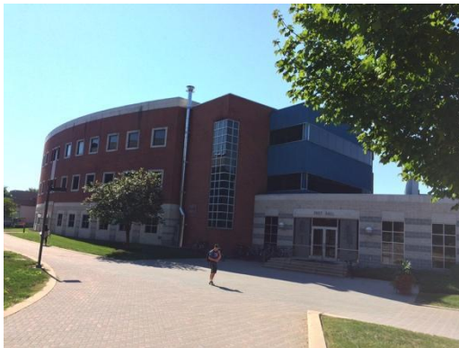
Frey Hall Hot water and chilled water
