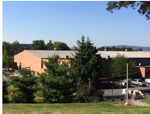
Eisenhower Campus Center & Sollenberger Sports Center Electricity, hot water, and chilled water
