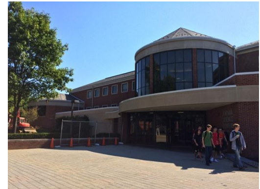
Kline Hall & Jordan Science Center Hot water and chilled water
