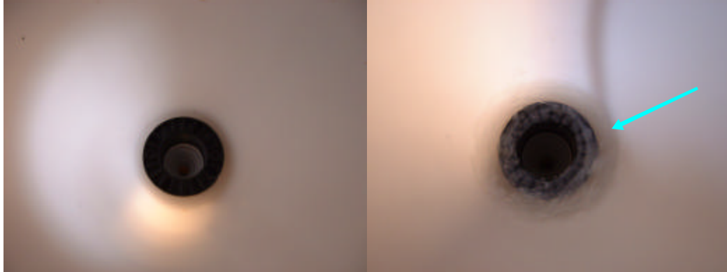
Figure 3.1.5 Bottom of RSW Tank before adding Silicon
